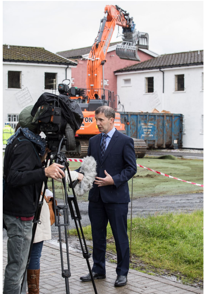
The Cabinet Secretary for Justice, Michael Matheson MSP visiting HMP & YOI Cornton Vale as demolition work gets underway
